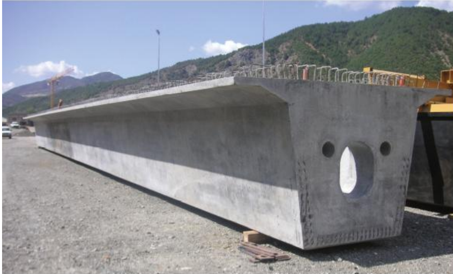
U SHAPE BEAM SELF REACTING MOULD
