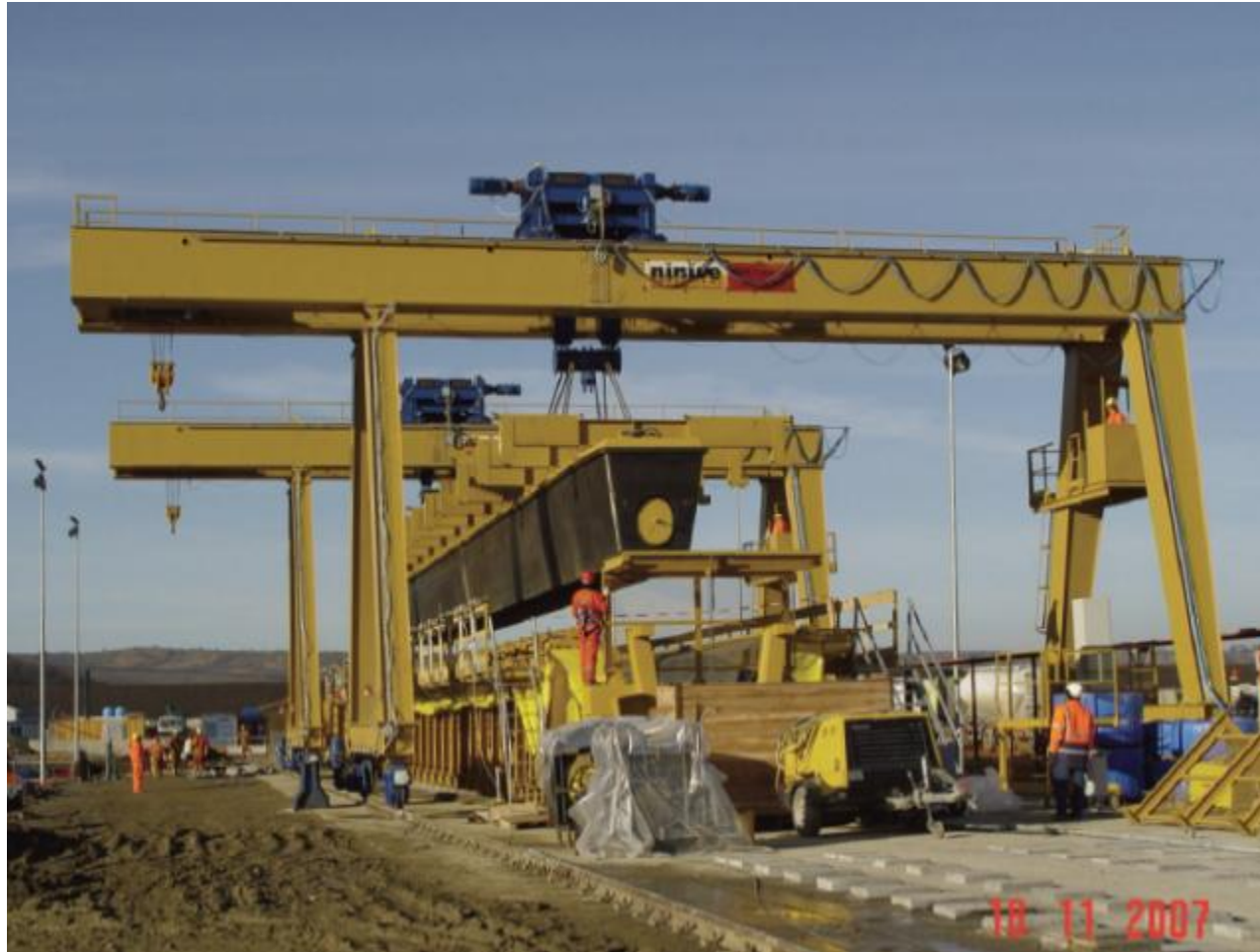
“U” SHAPE BEAM SELF REACTING MOULD
