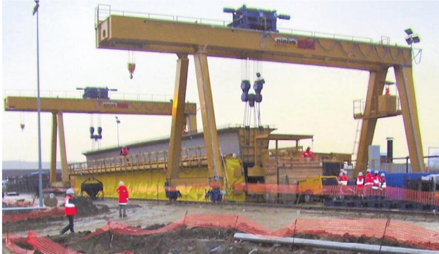
“U” SHAPE BEAM SELF REACTING MOULD
