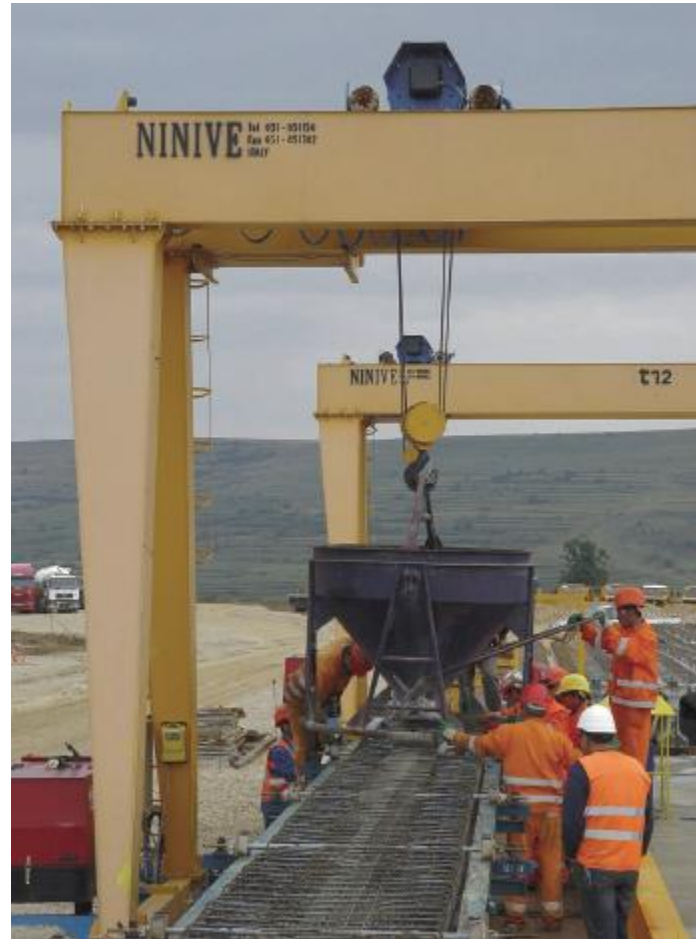
T” SHAPE BEAM SELF REACTING MOULD
